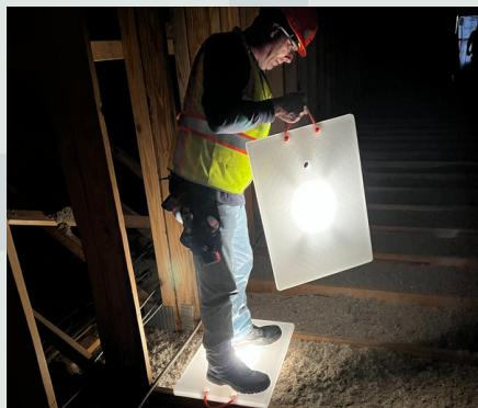
Position the next board at a comfortable distance. Step onto that board. Pick up and reposition the board you just vacated. Repeat to traverse the attic.
